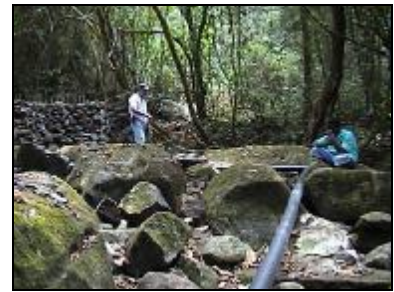
Tacugama dam and pipe system
