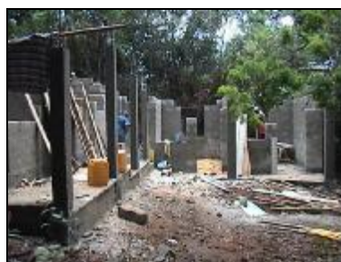
Construction of the new staff quarters
